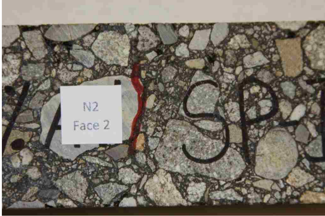
Figure 6.4 Fatigue Cracking in HMA Beam Sample SP-II-N2
