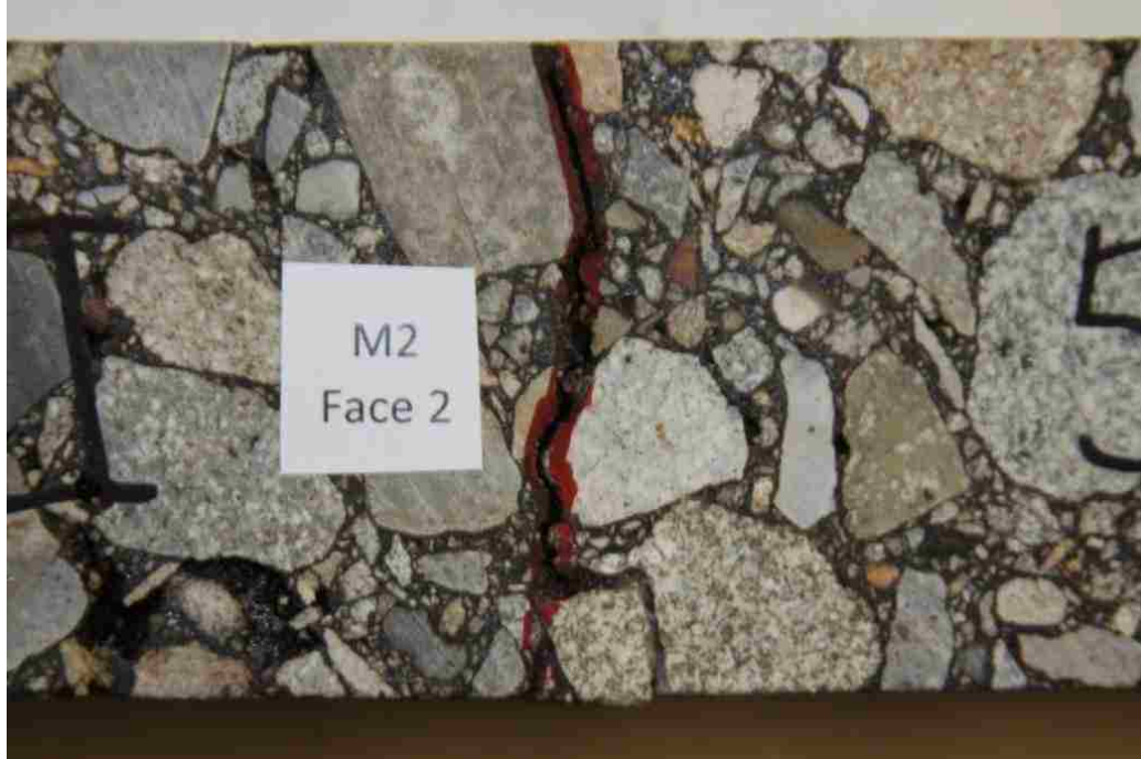
Figure 6.3 Fatigue Cracking in HMA Beam Sample SP-II-M2
